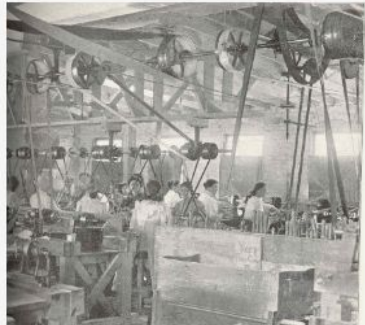
Drilling holes in buttons in the Mussel Fishery and Pearl-Button Industry
